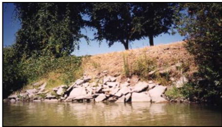
Channelization and bank stabilization
