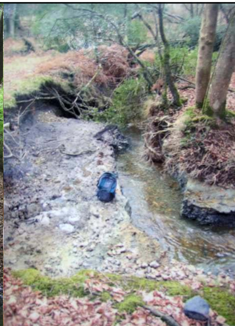
Highland Water. Structure ruined by poor management [2002]
