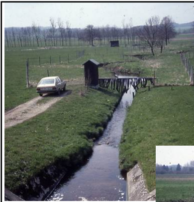
The Boyerbach, Bavaria One of many projects implemented by Walter Binder and co.
