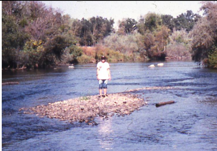
Gravel scoured and transported from constructed riffles after 4 drought years -Application of Shields' criterion shows the imported gravel was mobile at the post-dam Q1.5
