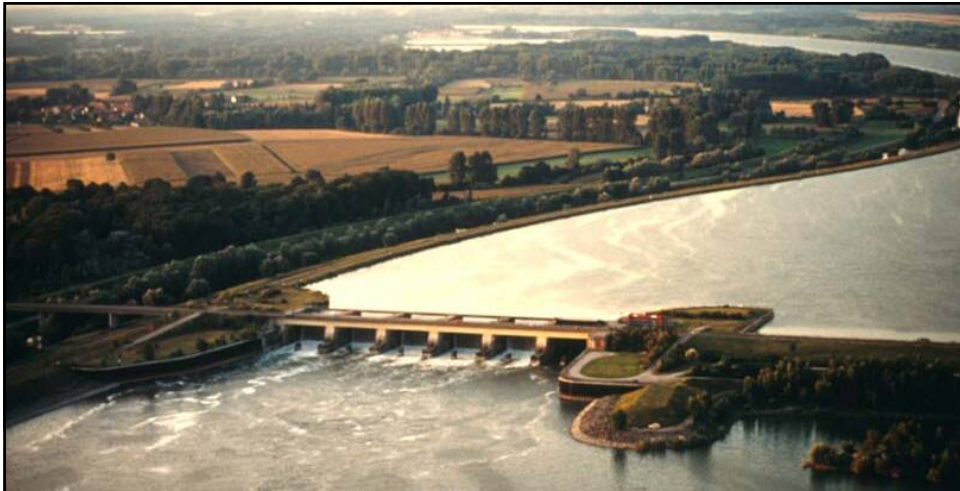
Iffezheim: the downstream-most dam
