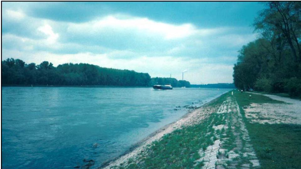
Gravel augmentation on the Rhine: to prevent undermining of infrastructure
