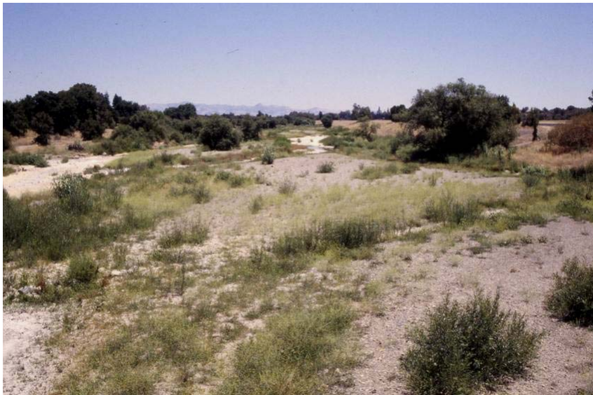
Uvas Ck (same view as last photo) July 1997 Channel failed Feb 1996, 3 months after construction
