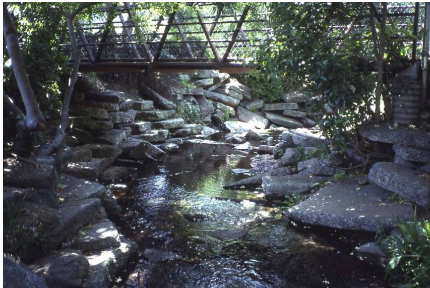
“Daylighted” channel of Strawberry Creek, banks formed by concrete rubble from destroyed culvert
