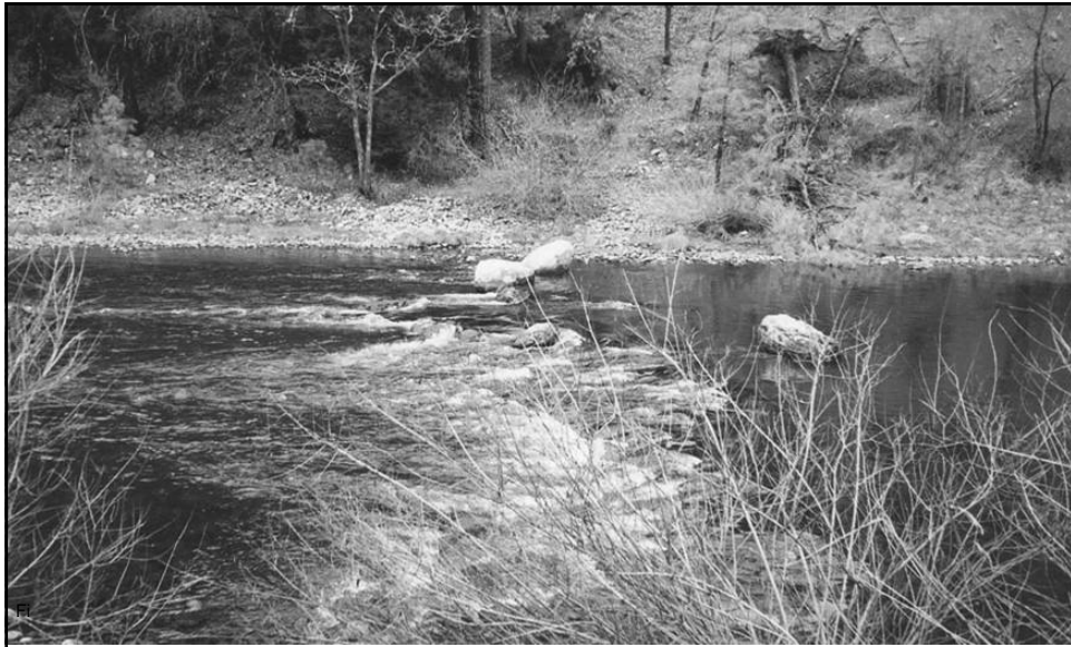
Artificial riffles designed to create spawning habitat by creating the forms
