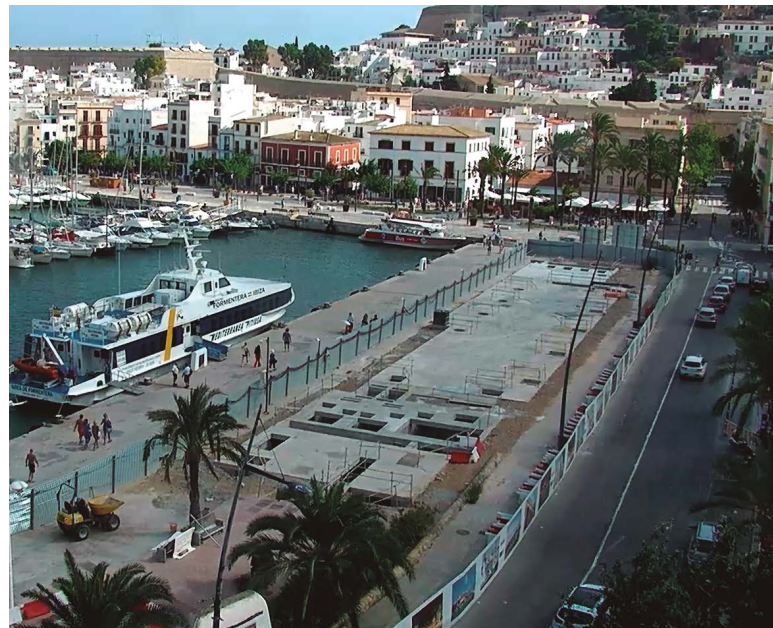
Ibiza storm tank (Balearic Islands)
