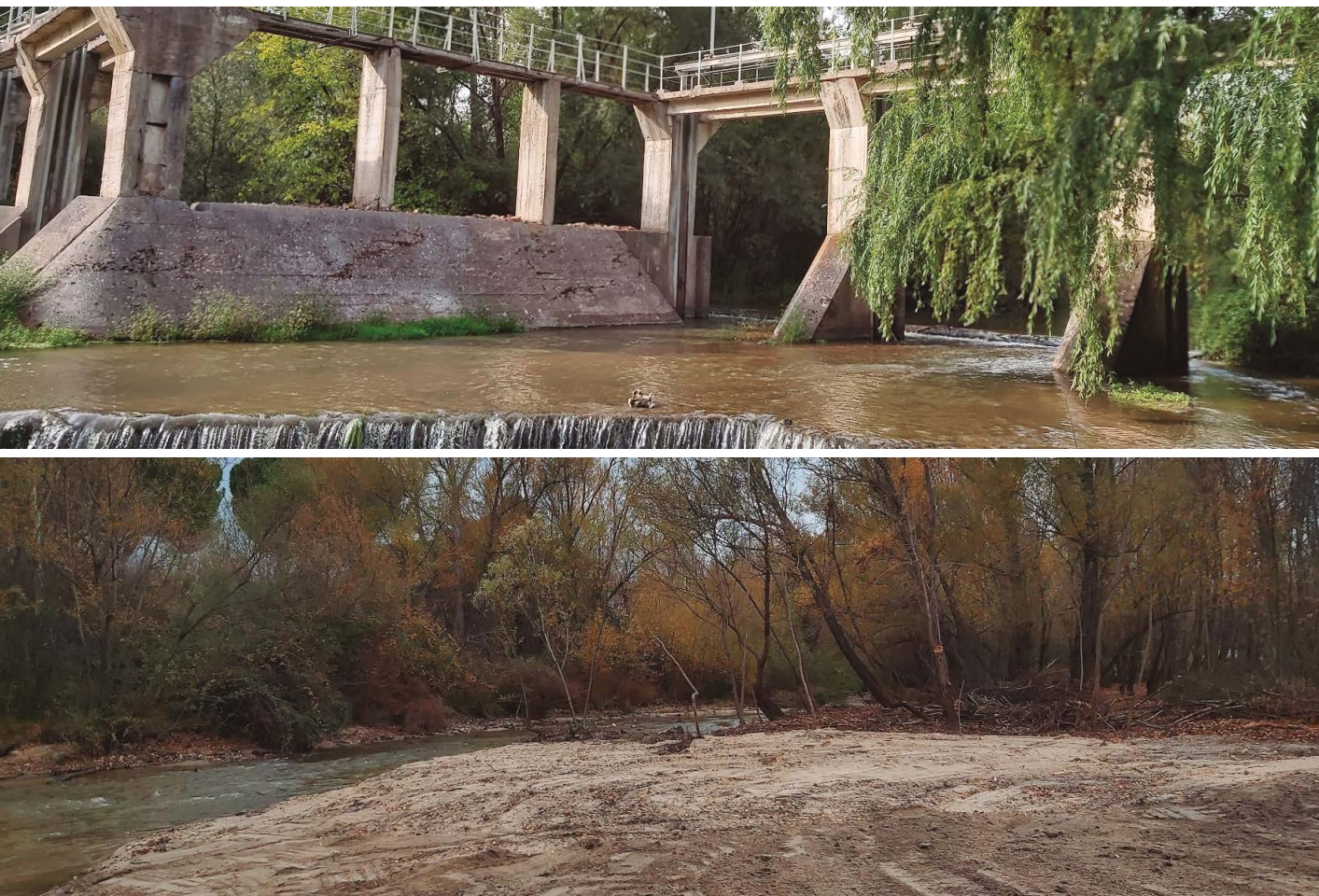
In the first image, an obsolete weir in the Manzanares river, Tajo basin, in El Pardo (Madrid). In the second image, the weir has already been removed
