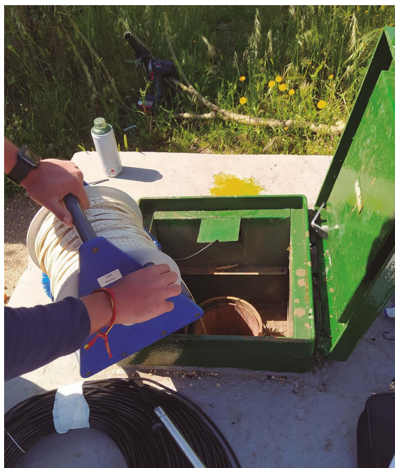
Manual measurement of the groundwater level
