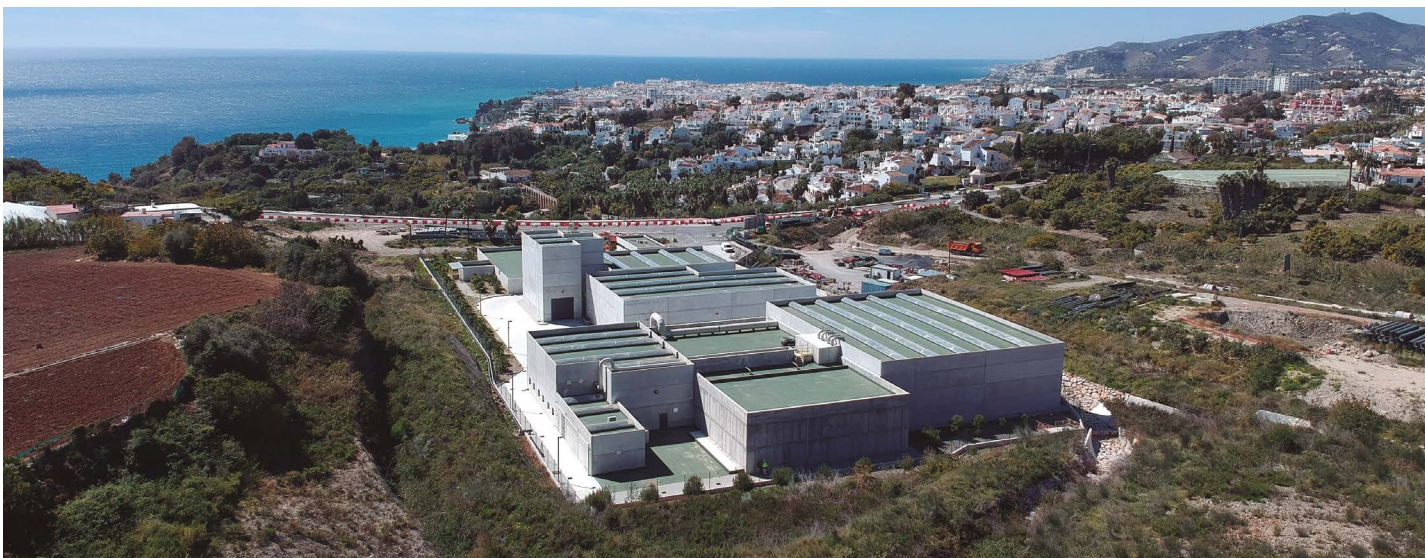
Nerja WWTP, Andalusian Mediterranean Basins (Málaga, Andalusia)
