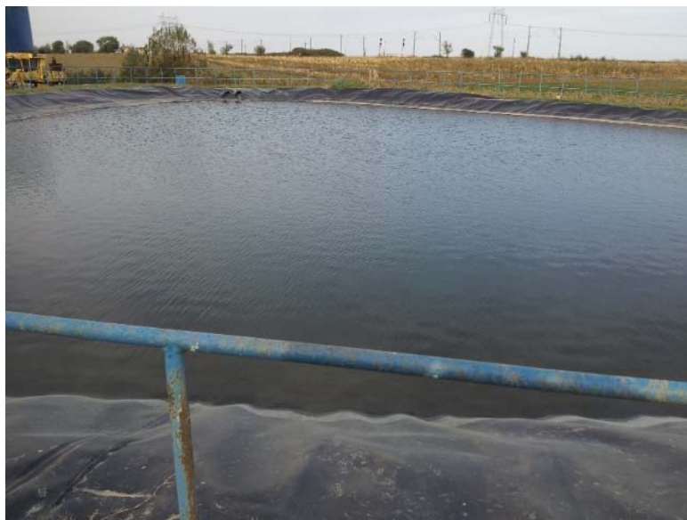
Figure 25: Lagoon for treated leachate water at Landfill in Romania
