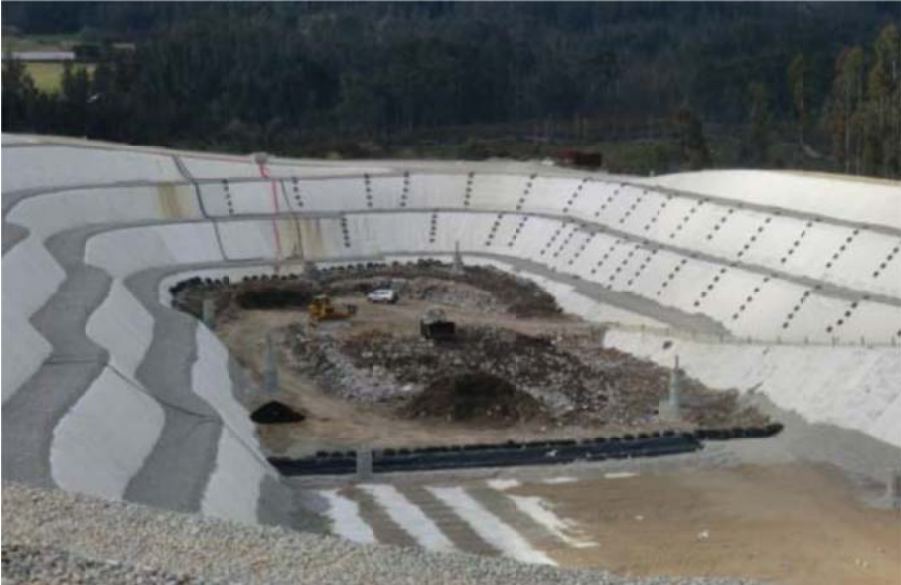
Figure 46: Cell construction
