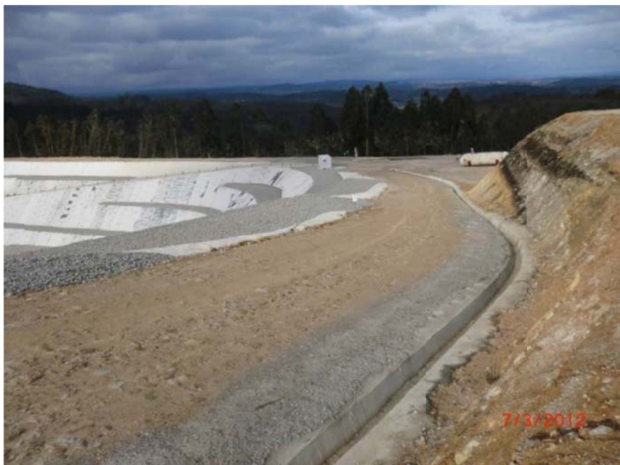
Figure 49: Ditch perimeter of rainwater
