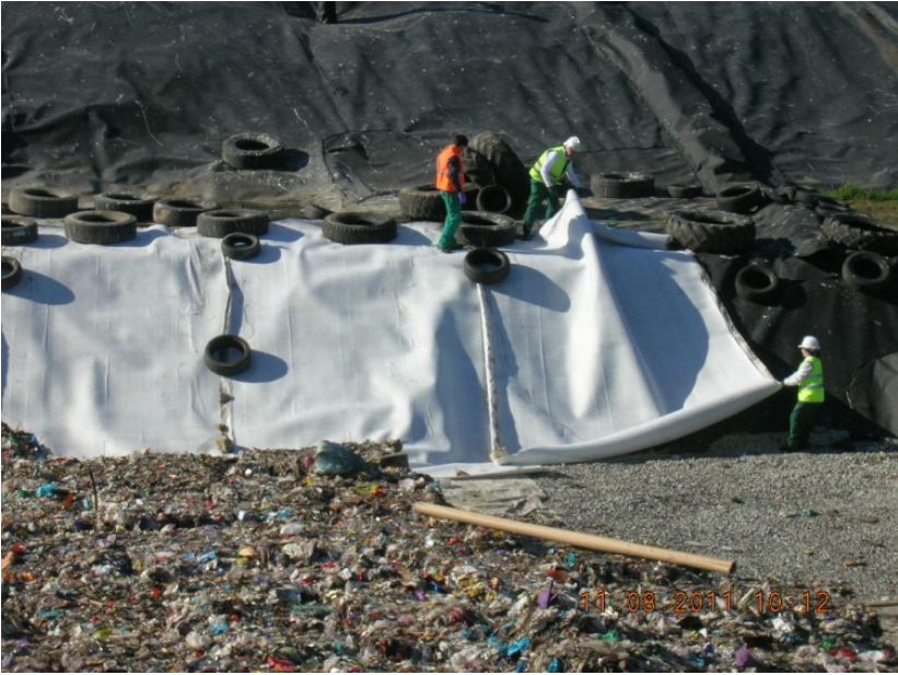
Figure 52: Attaching the composite drainage
