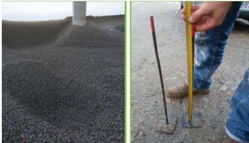
Figure 42: Thickness of gravel layer
