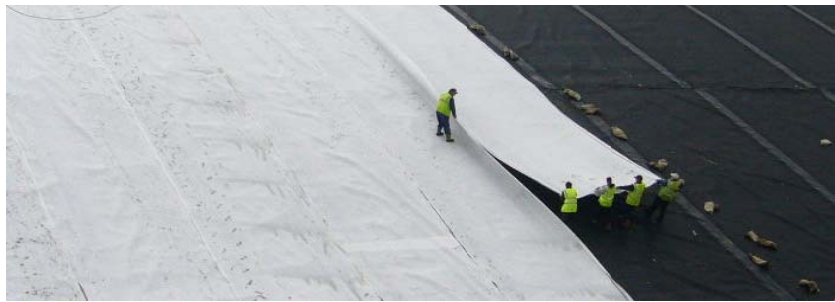
Figure 44: Preparing the bottom - materials
