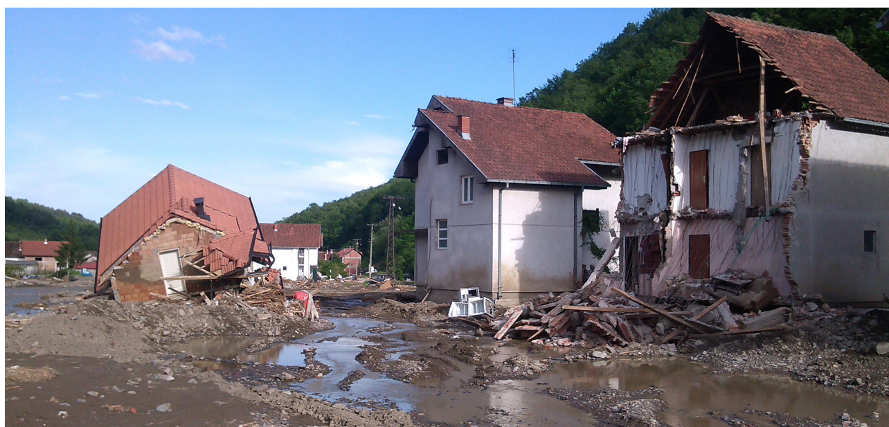
Figure 3.2 Flood and mudslide damage to houses in the town of Krupanj, Serbia, 2014
