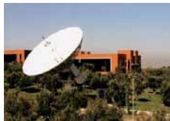
Ground Segment infrastructure
