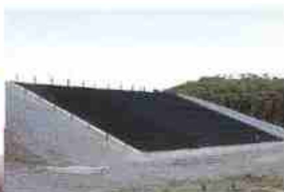
Field tests of sheet lining
