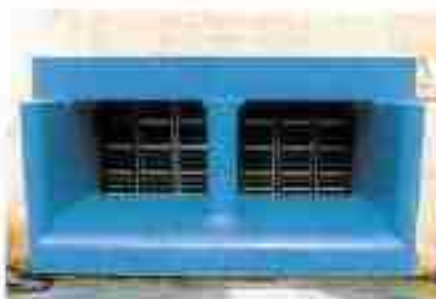
Surface coating of the outlet and FRP screens
