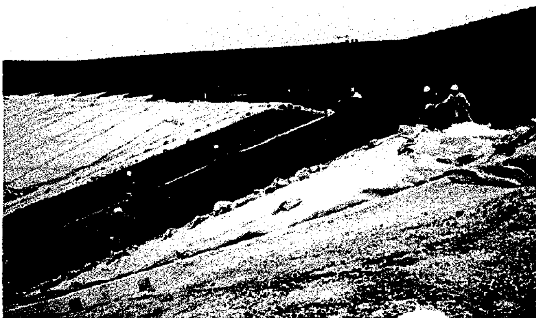
Photo 4. Rubber sheet installation
